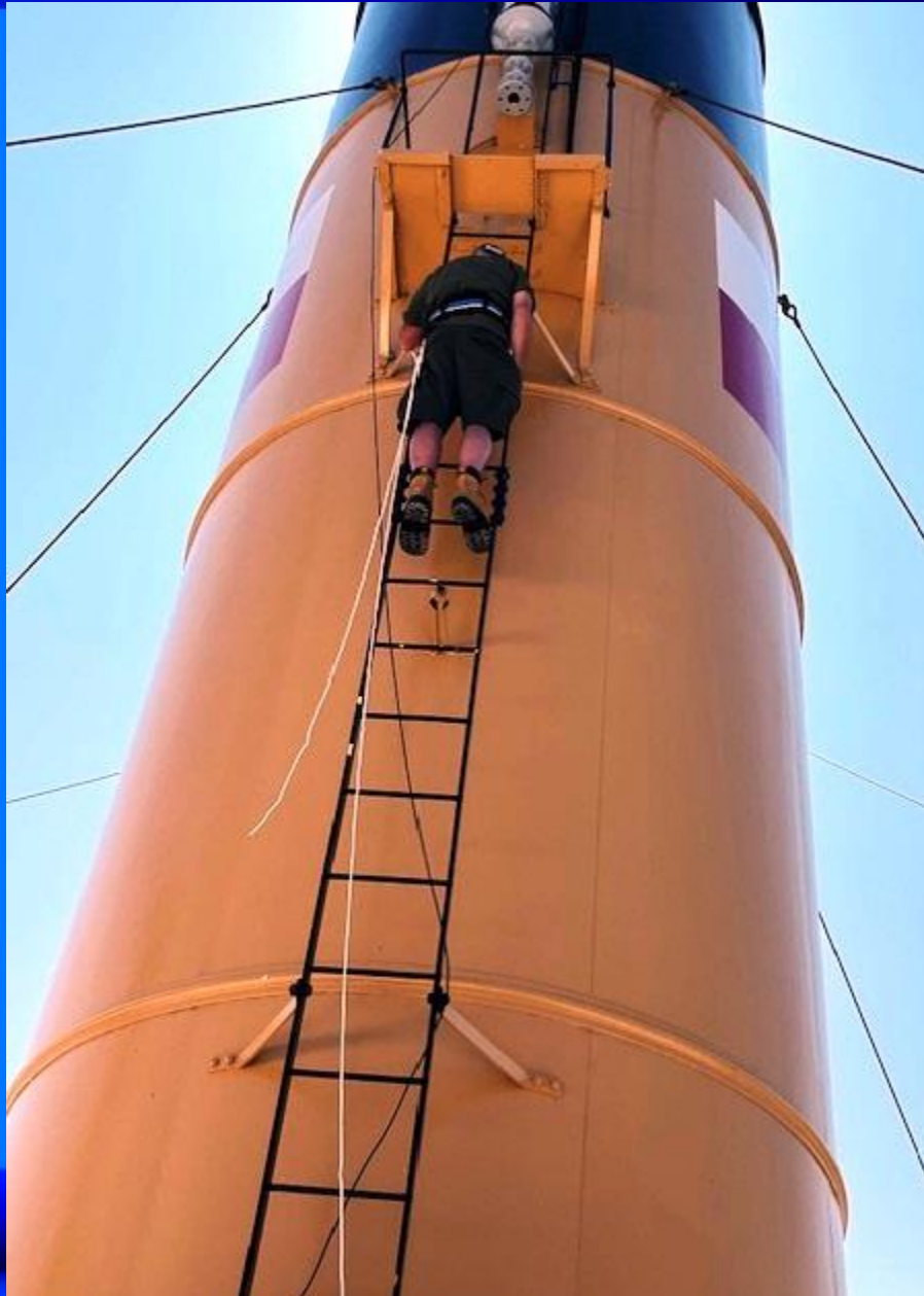
Hardware for the aft end of the HF antenna being installed on Keewatin's funnel
