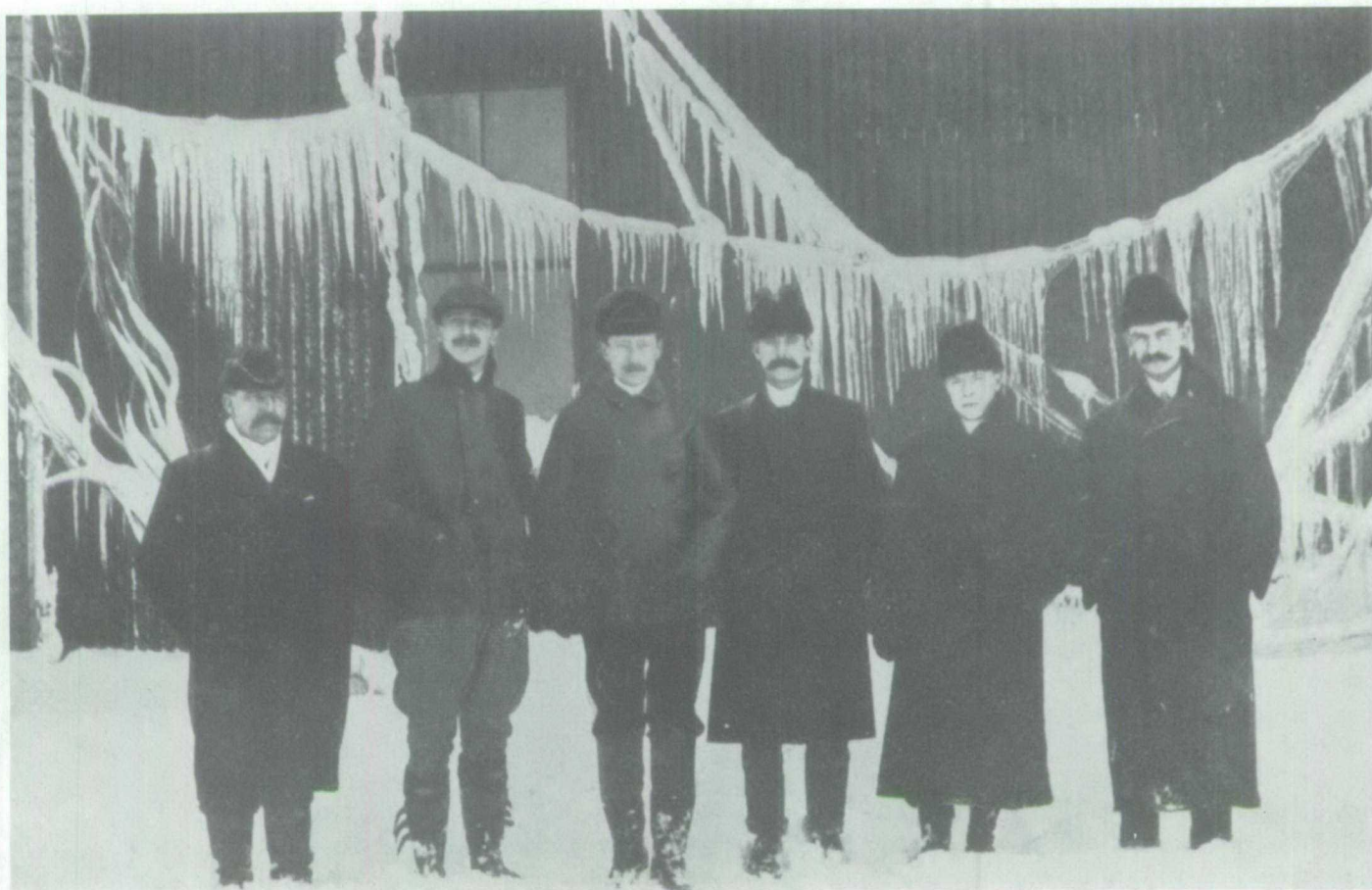
Marconi and his staff outside the transatlantic station at Glace Bay, Nova Scotia. The men are standing in front of an antenna brought down by a heavy coating of ice, 6 April 1903. Source: R.N. Vyvyan, Wireless Over Thirty Years (London: George Routledge & Sons, 1933)
